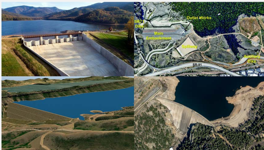
FIGURE 2-3 Example dam projects that use PMP for rehabilitations, expansions, and new designs (clockwise from upper left): North Fork Dam, Prado Dam, Gross Dam, Chimney Hollow Dam. SOURCE: City of Asheville; USACE (2021); Mitch Tobin/WaterDesk.org, with aerial support provided by Lighthawk; Northern Water.
