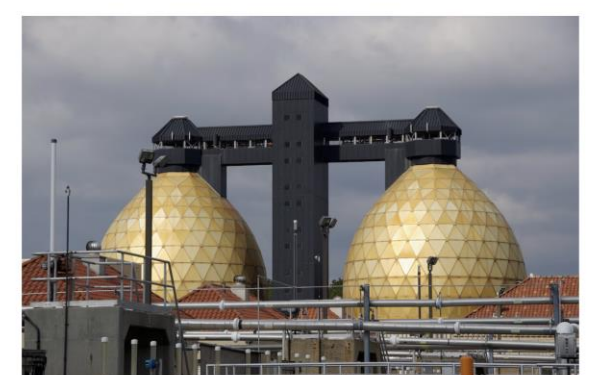
The two digesters at the Back River Wastewater Treatment Plant near Baltimore. (Kristian Bjornard/Wikimedia)
